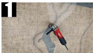
Crack Surface Prepare
