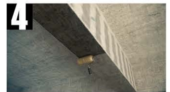
Applying Carbon Epoxy
