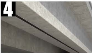
Placement of CFRP Plates
