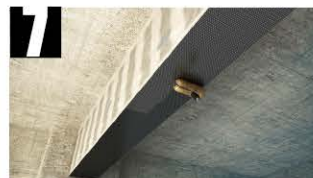
Applying Carbon Epoxy Again
